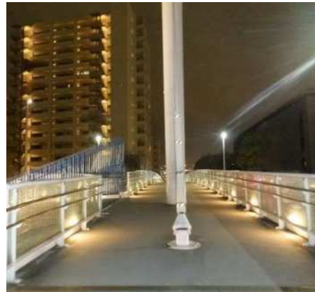
灘の浜歩道橋高欄照明LED化(R4.3完了)
